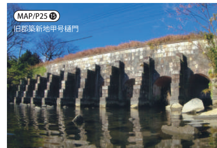
Former Gunchiku-Shinchi Kogo sluice gate
